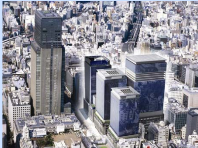
Muromachi East District Development Project Blocks 2-5, 1-5 (2013)
