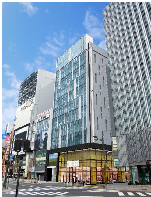
An external view of Shinjuku M-SQUARE
