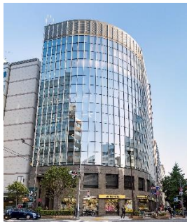
New hub (Tosho Building)
