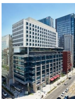
OVOL Nihonbashi Building
