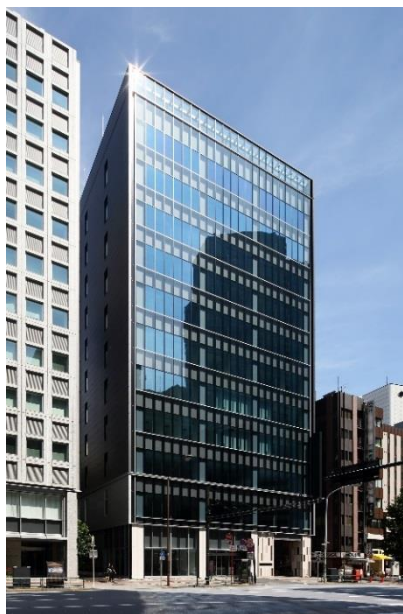
Exterior view of Shinbashi M-SQUARE Bright
