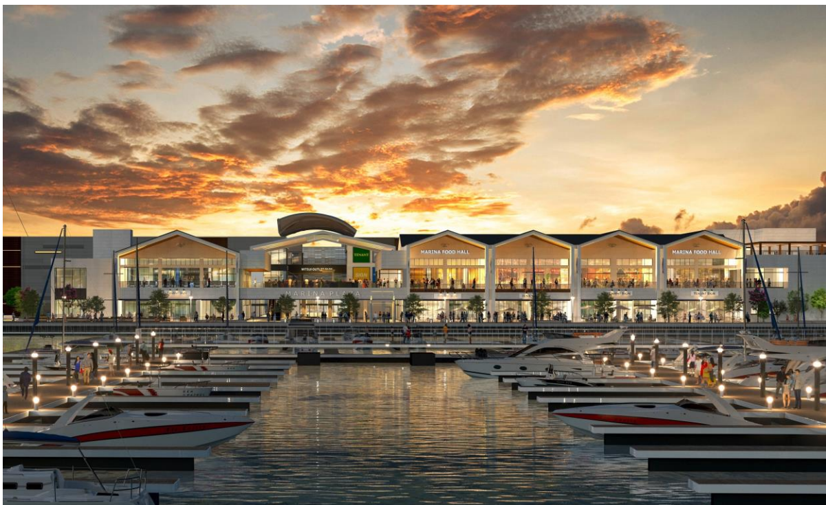
Exterior Image (southeast side)
