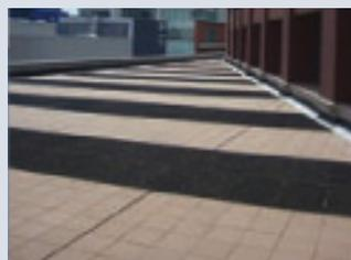
Water retaining panels installed on the roof use a sprinkling effect to help cool the building.
