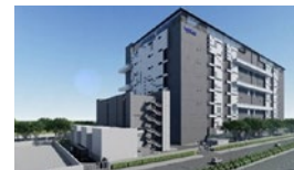
(仮称)CapitaLand DC Mumbai
