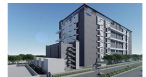
(仮称)CapitaLand DC Mumbai
