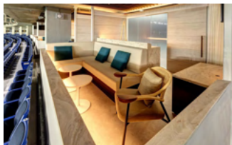
魅力溢れる観客席の新設 Installation of attractive seating
