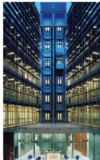
Projects @ Hopkins Architects GEK Group Headquarters
