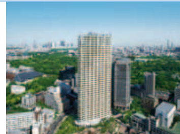
Park Court Akasaka The Tower
