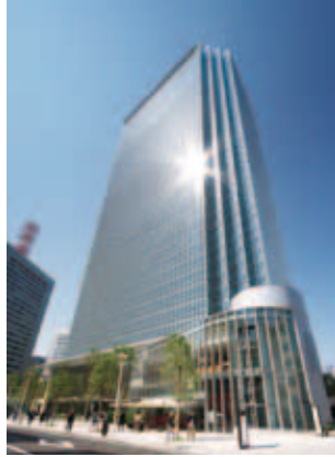
Akasaka Biz Tower (Completed in 2008 / 218,000m 2 )
