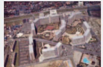
Chiba Garden Town (Completed in 1975)
