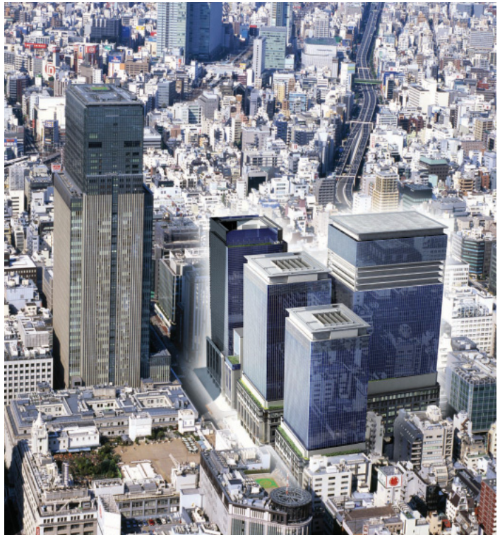
Nihonbashi Muromachi East District Development Projects
