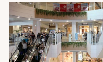
Adoption of a Co-generation System At Lalaport Ebina, a cogeneration system has been deployed that produces and supplies electric power and heat simultaneously, and is used in air conditioning and other systems
