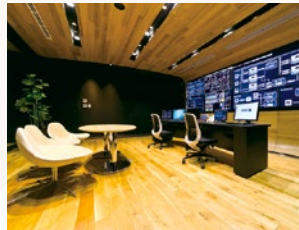
Kashiwa-no-ha Smart Center district energy operations base
