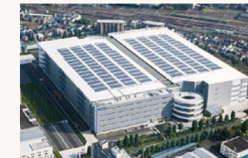
Installing Solar Power Equipment At MFLP Hino, in addition to installing a solar power system with a generating capacity of approximately 2 MW, energy-saving performance is enhanced through the use of LED lighting throughout the facility and other measures
