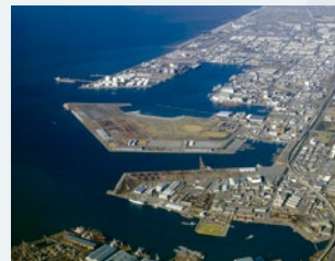
Keiyo rinkai reclamation project, Chiba Prefecture (late 1950s)
