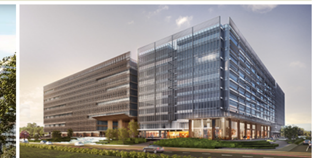
RMZ Ecworld 30 (Bangalore, India) Phase 1 to be completed in 2022/Phase 2 to be completed in 2023
