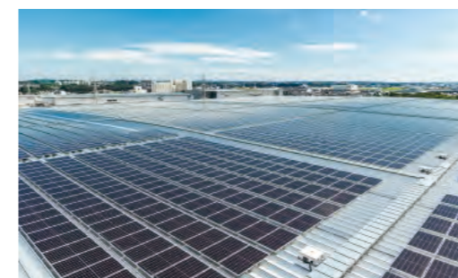
Solar panels installed on the rooftop
