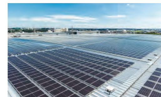
Solar panels installed on the rooftop
