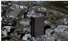
1968 Developed the Kasumigaseki Building (Contributed to the accumulation of urban functions)
