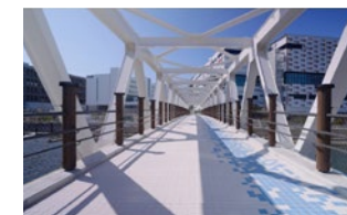
Developing Azora Bridge to promote pedestrian traffic (MFIP Haneda)
