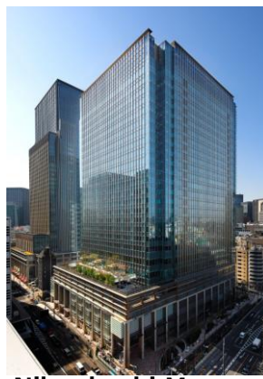
Nihonbashi Muromachi Mitsui Tower (Tokyo, 2019)
