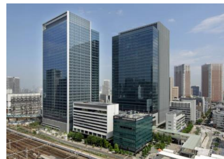
msb Tamachi (S and N buildings) (Tokyo, 2018 and 2020)
