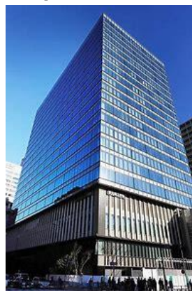
Bunkyo Garden Gate Tower (Tokyo, 2020)
