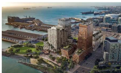
Mission Rock / San Francisco Housing Office
