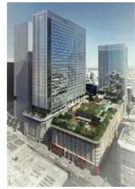
Nihonbashi Takashimaya Mitsui Building (Completed in 2018)
