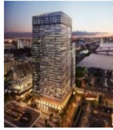
TOYOSU BAYSIDE CROSS (Completed in Mar. and Oct. 2020)
