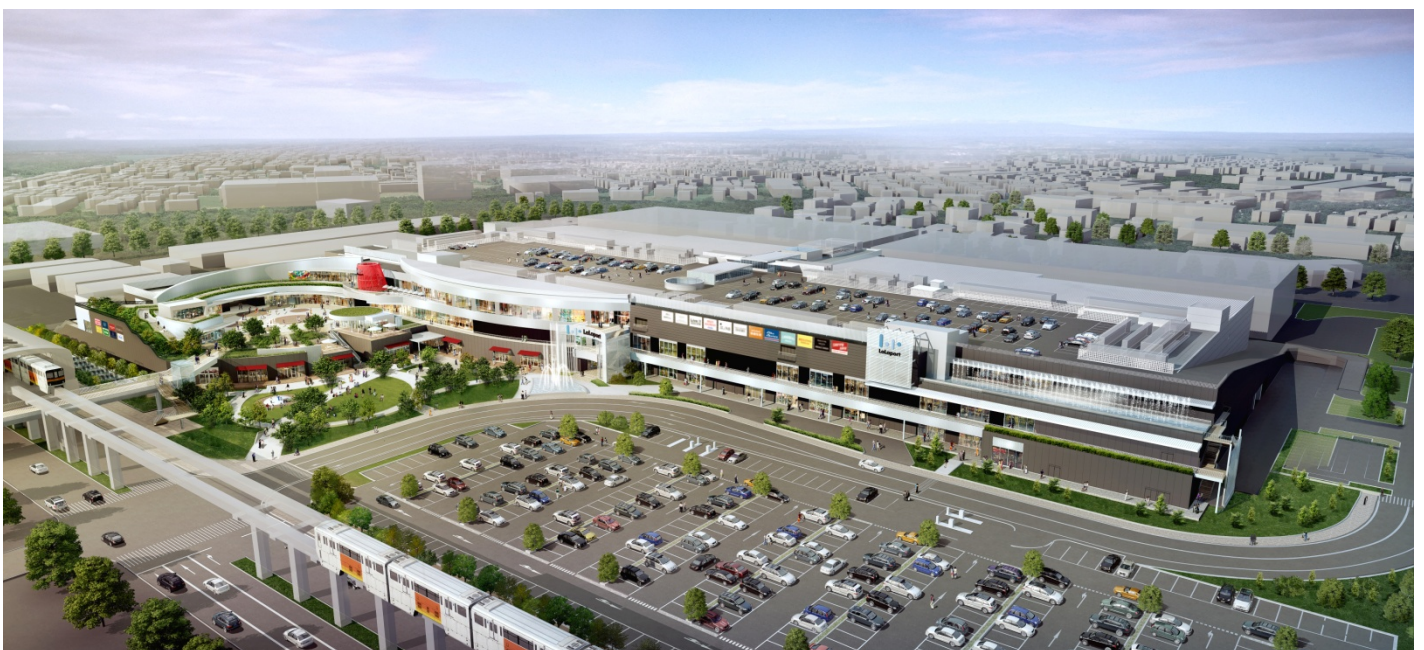
External view of the facility
