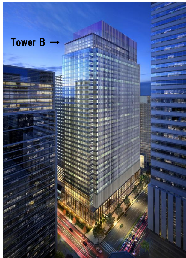
View of Tower B from the Hibiya-dori Street side
