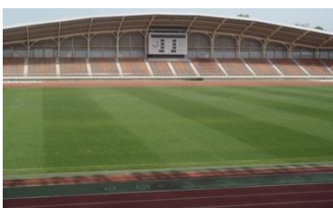
Sports stadium in Kashiwanoha
