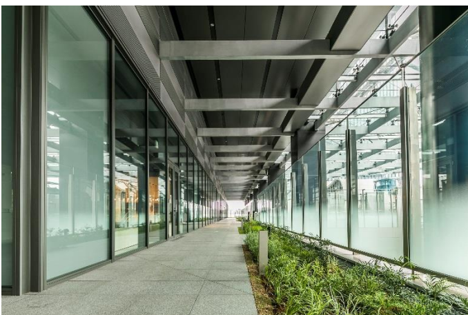
Zone C Rooftop Garden
