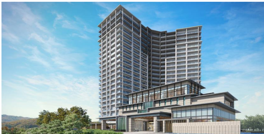
CG image of the completed PARK WELLSTATE Kamogawa Project (tentative name)
