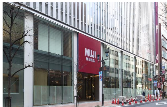
Exterior view of the lower floor of Yomiuri Namiki-dori St. Building
