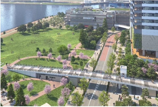
Toyosu Park Bridge provides access to Toyosu Park
