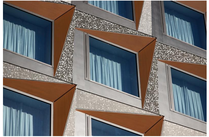
Exterior wall with wood grain pattern
