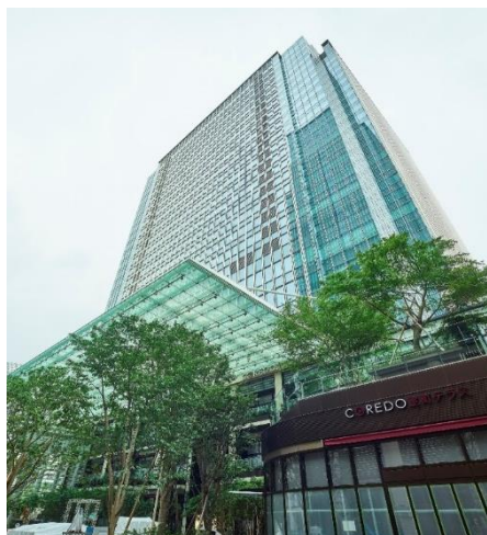
Exterior of Nihonbashi Muromachi Mitsui Tower
