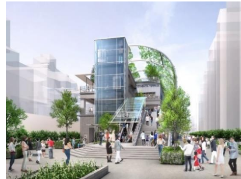
Computer generated image of the South Block entrance of MIYASHITA PARK
