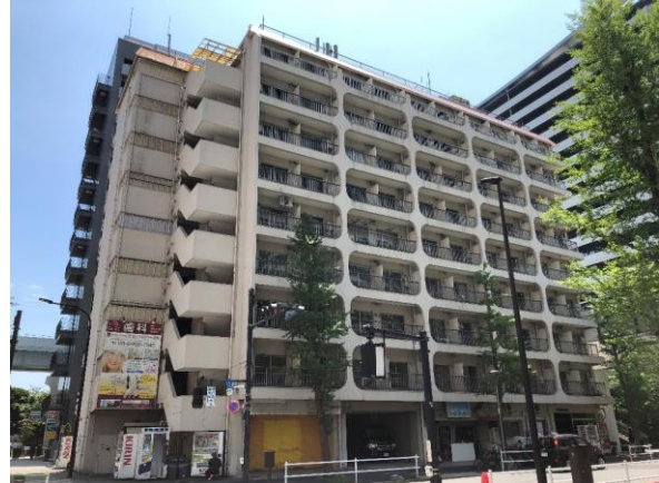
[ Exterior view of the property before rebuild ]
