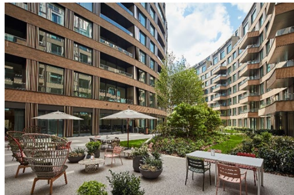
Residential housing inside the Television Centre Redevelopment Project
