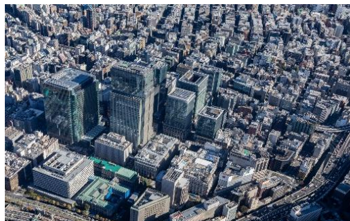
Nihonbashi Smart Energy Project
