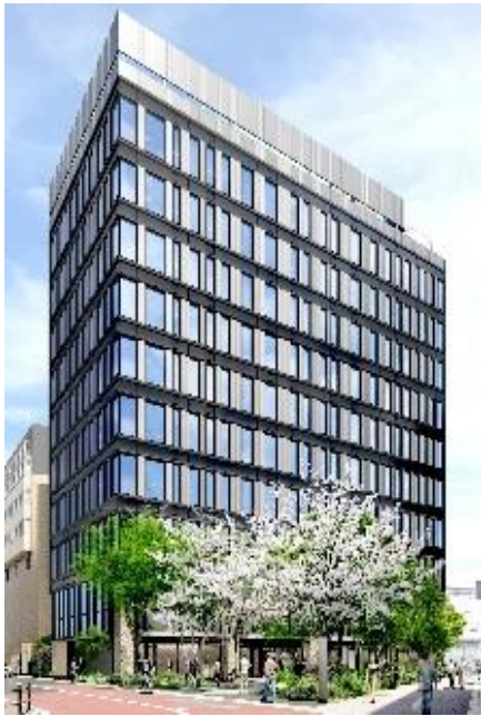
Tamachi M-SQUARE Garden (ZEB Ready)
