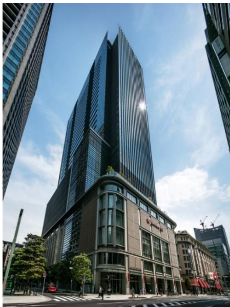
Nihonbashi Takashimaya Mitsui Building exterior
