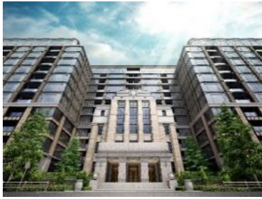
Façade (South side entrance)
