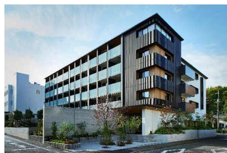
Timber condominium MOCXION
