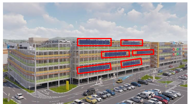
Multi-story parking building Computer generated image of solar panels installed in a wall (areas with a red border are solar panel installations)
