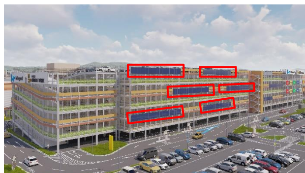
Multi-story parking building Computer generated image of solar panels installed in a wall (areas with a red border are solar panel installations)
