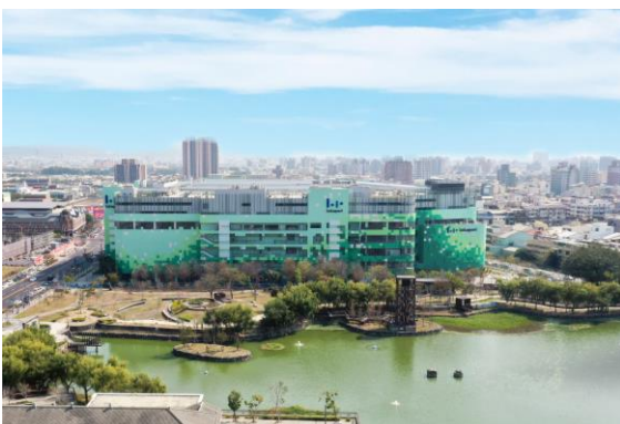
Exterior view of the North Building
