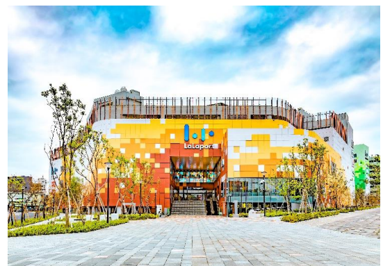
Exterior view of the South Building
