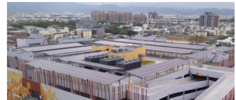
Solar panels on the roof of the South Building
