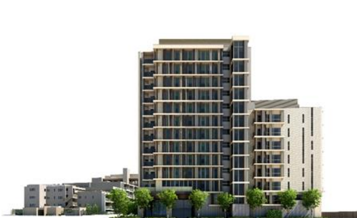
CG image of completed exterior
