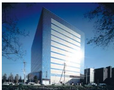
Exterior view of Shinkiba Center Building
