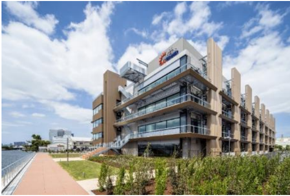
Exterior view of MITSUI LINK-Lab SHINKIBA 2 (southeastern side)
