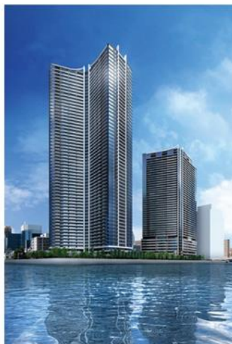
Park Tower Kachidoki Mid/South
