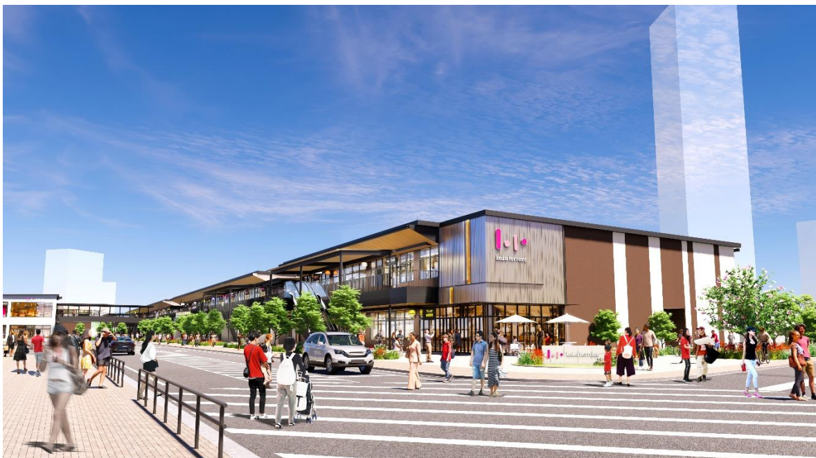
Conceptual image of the exterior of Mitsui Shopping Park LaLa Terrace TOKYO-BAY
