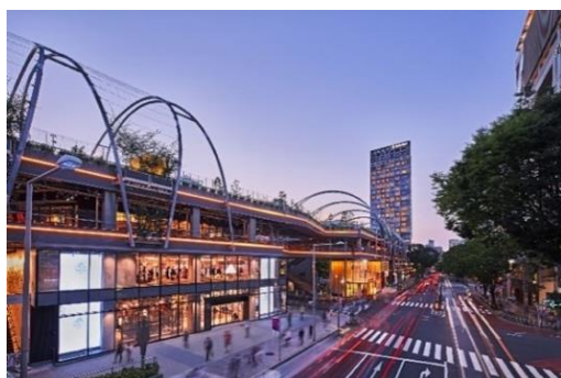
MIYASHITA PARK external view
