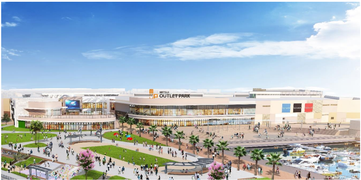
Computer generated image of the exterior of MITSUI OUTLET PARK MARINE PIA KOBE Reconstruction Project
