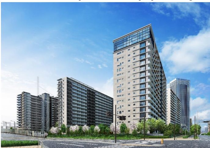
CG illustration of completed exterior
