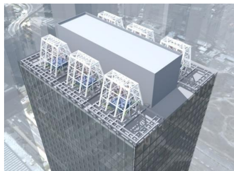
Schematic of the Shinjuku Mitsui Building ultra-large vibration control device
